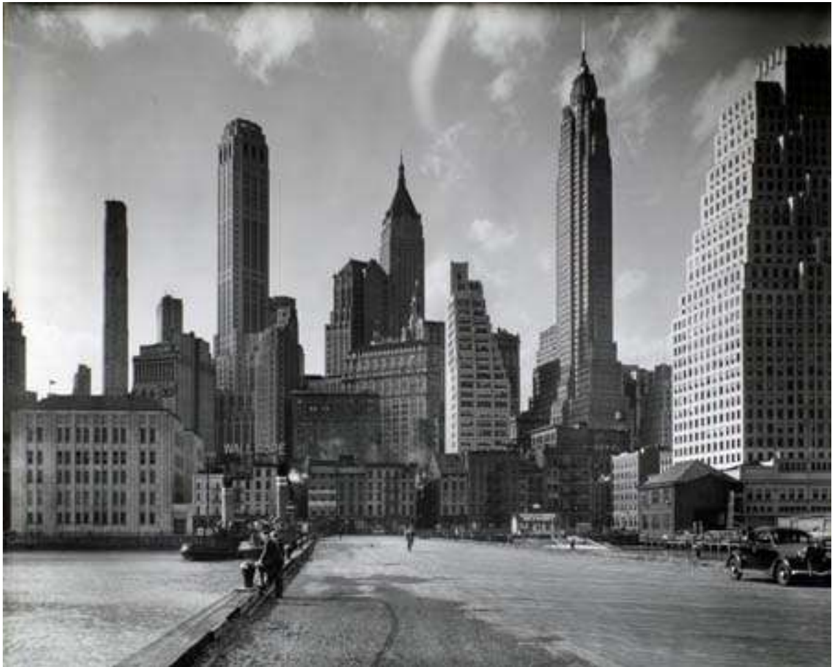
Manhattan, Skyline I South Street and Jones Lane - Manhattan by Berenice Abbott, March 26 1936
